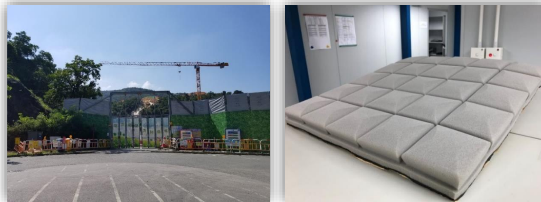
圍街板加設隔音棉
